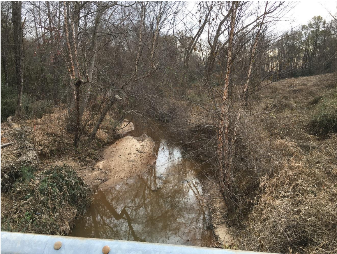
Looking downstream from Honbarrier Drive Bridge over Rocky Creek.
