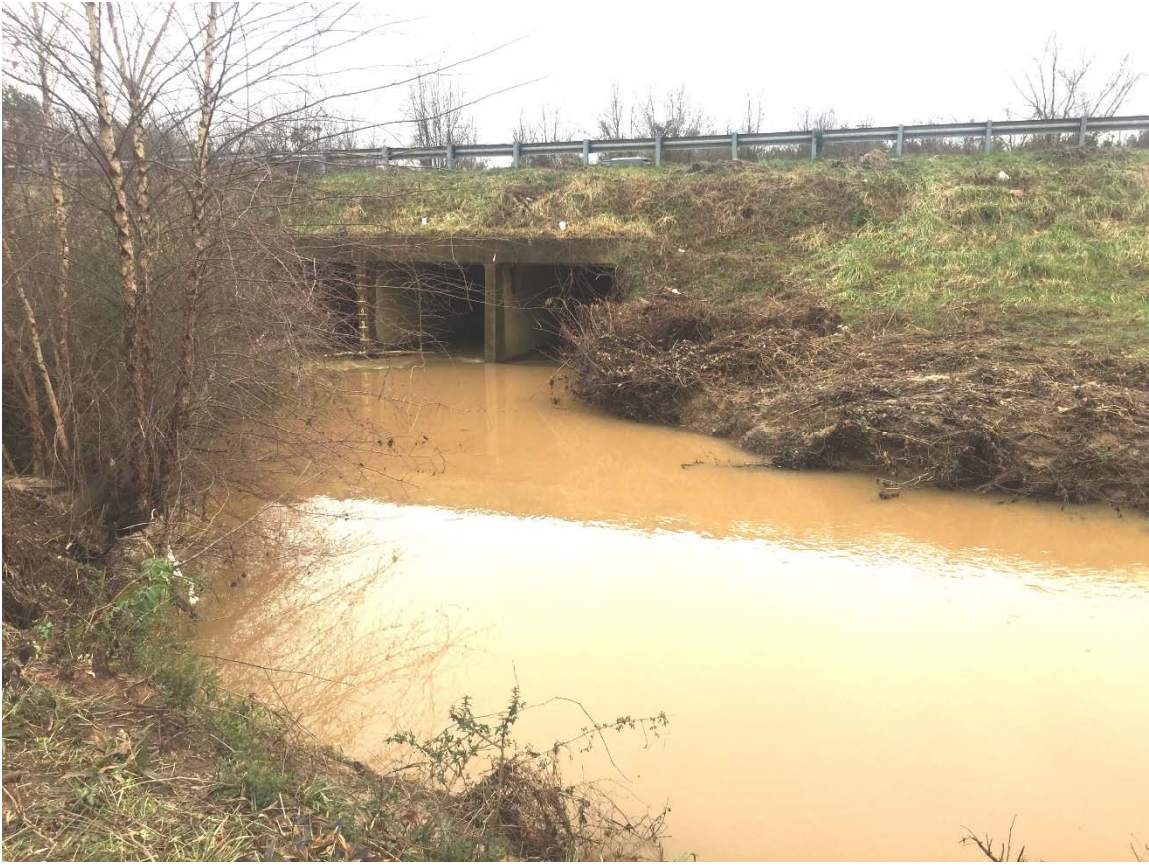
Looking downstream at I-85 box culverts at Rocky Creek
