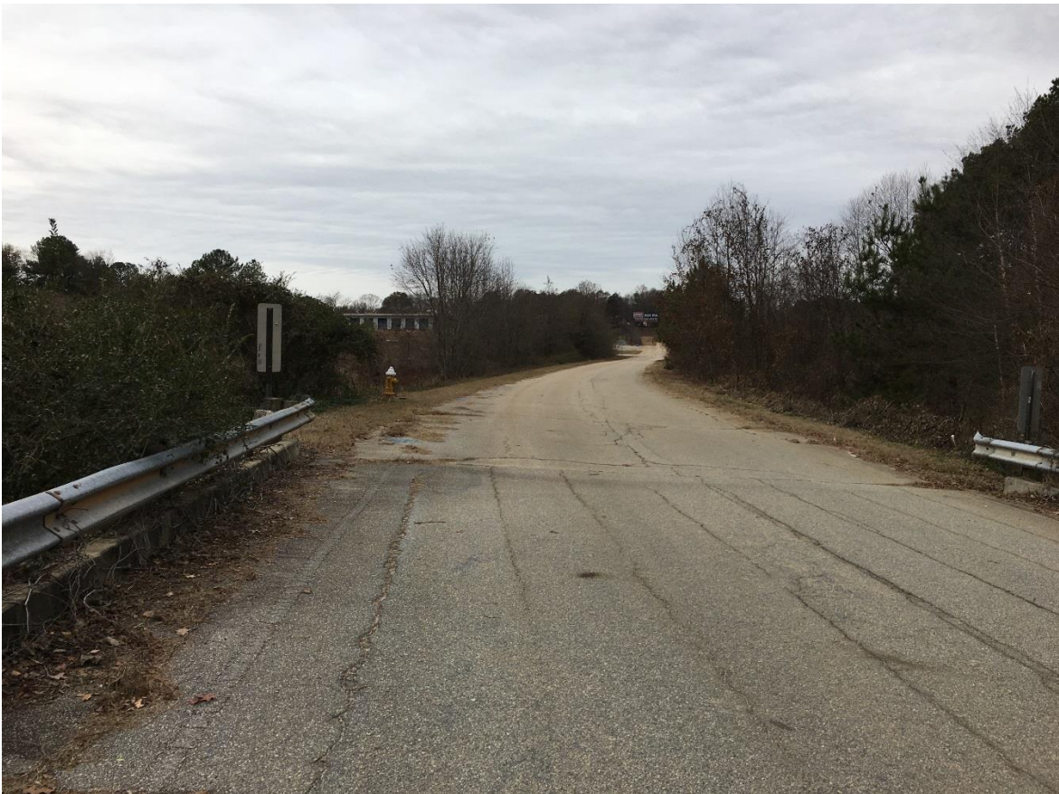
Looking west from Honbarrier Drive Bridge over Rocky Creek.
