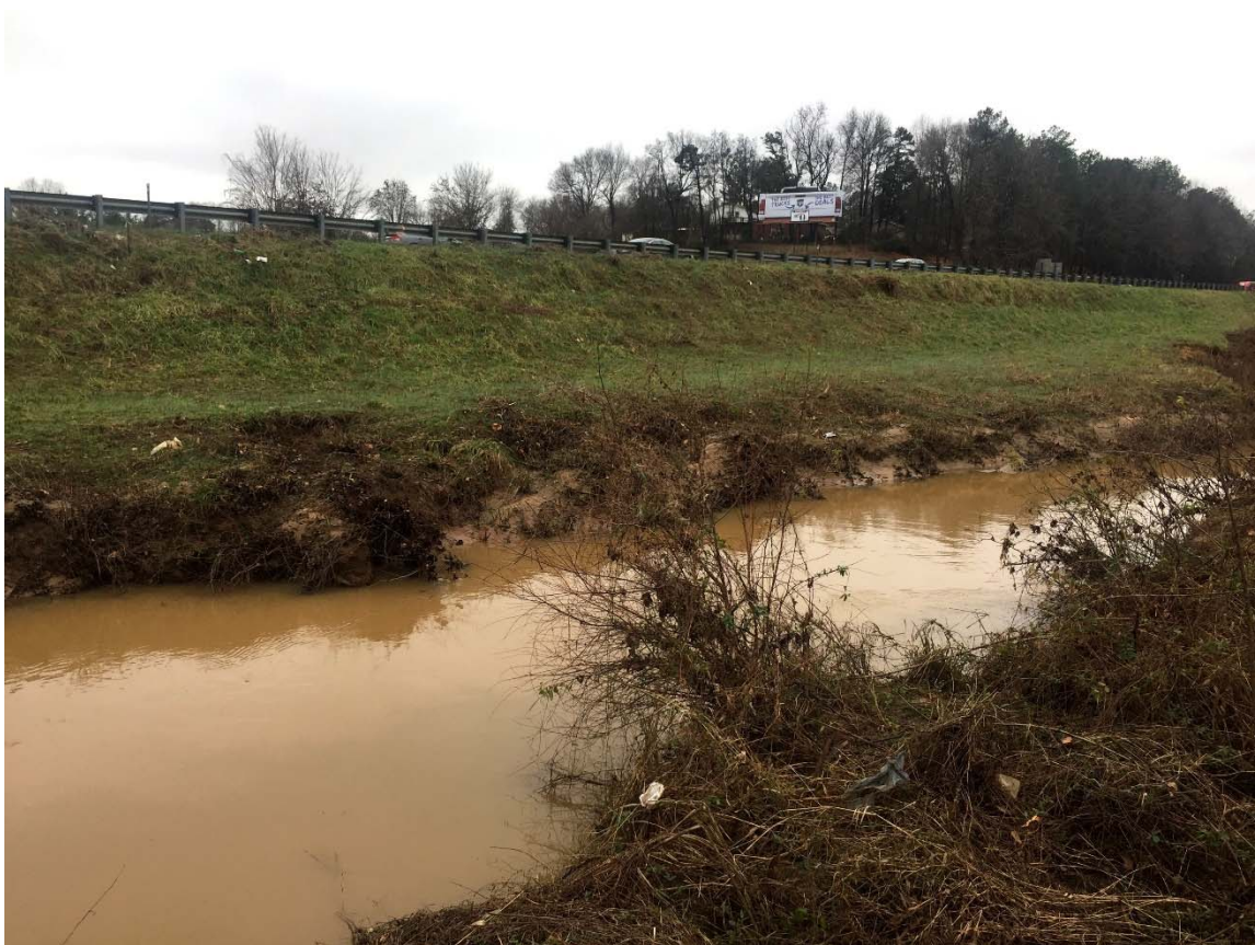
Looking upstream of I-85 box culverts
