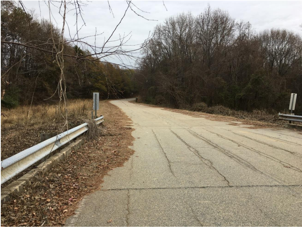
Looking east from Honbarrier Drive Bridge over Rocky Creek.
